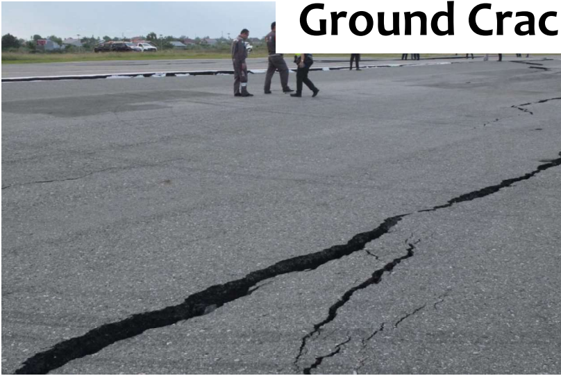
Ground Cracking at Palu Airport
